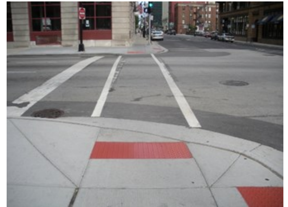
ADA Compliant Sidewalk Ramp
