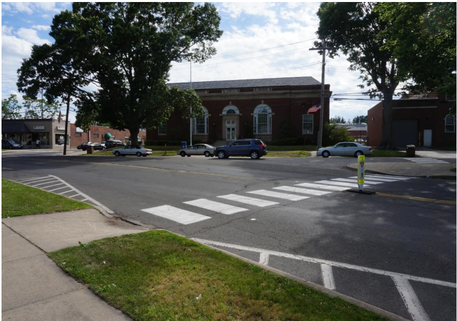
USPS on River Street
