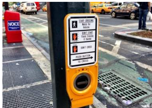
Accessible Pedestrian Signal Push Button
