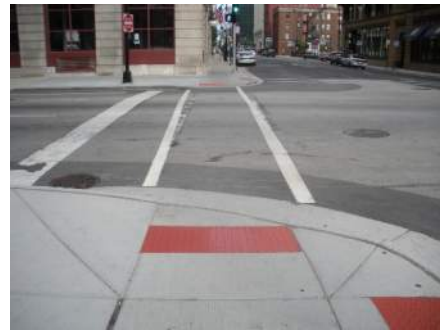
ADA Compliant Sidewalk Ramp
