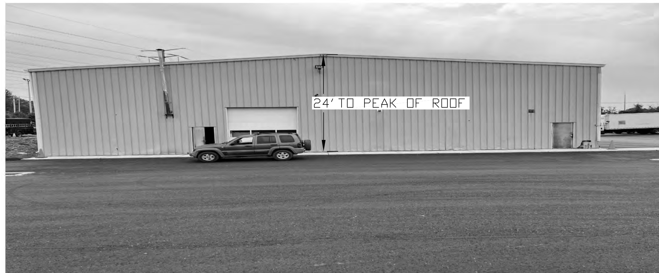
EAST SIDE--VIEW FROM PARKING AREA
