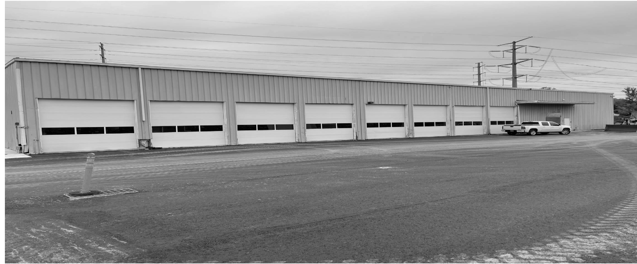
NORTH SIDE—VIEW FROM PARKING AREA
