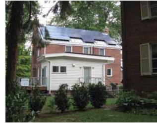
Not Recommended: [75] Solar roof panels have been installed at the rear, but because the house is situated on a corner, they are highly visible and negatively impact the character of the historic property.
