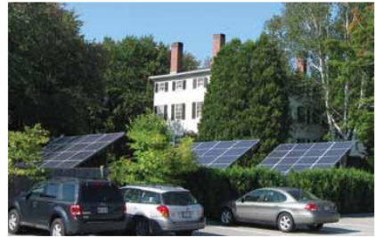
Not Recommended: [79] Although installing solar panels behind a rear parking lot might be a suitable location in many cases, here the panels negatively impact the historic property on which they are located.
