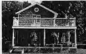
Address: 5 Center St. Owner: KIMBALL Style: Cottage Year built: 1880 Parcel no: 54 403 12
