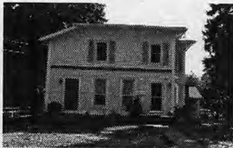
Address: 16/18 Union St. Owner: PISELLI Style: Vernacular Year built: 1915 Parcel no: 44 408 10
