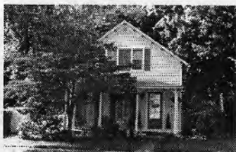
Address: 79 Lafayette St. Owner: SANDERSON Style: Cottage Year built: 1890 Parcel no: 44 410 8
