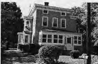
Address: 55 Lafayette St. Owner: McGUIGAN Style: Italianate Year built: 1900 Parcel no: 44 410 13
