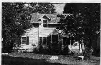
Address: 110 Lafayette St. Owner: MAZZEO Style: Cottage Year built: 1930 Parcel no: 44 408 11
