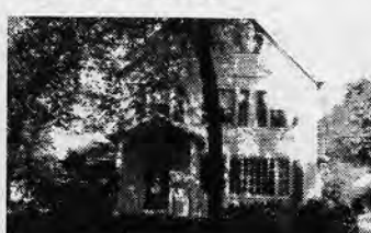
Address: 42 Green St. Owner: NORTHROP Style: Vernacular Year built: 1840 Parcel no: 44 406 5
