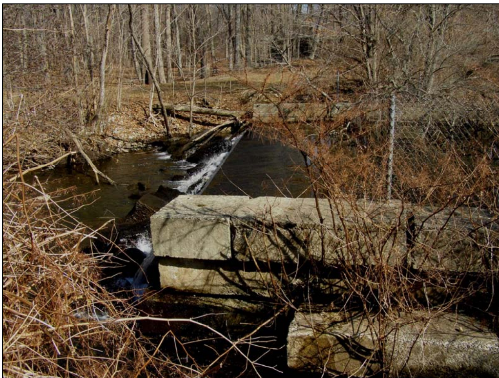
Dam at the outlet of the unnamed pond.
