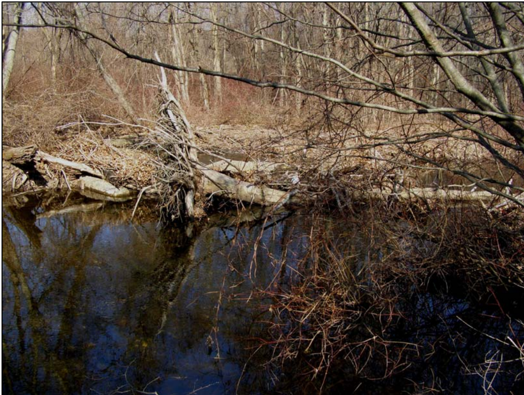
The diversion structure in the Wepawaug River. View of the structure is partially obstructed by fallen trees.
