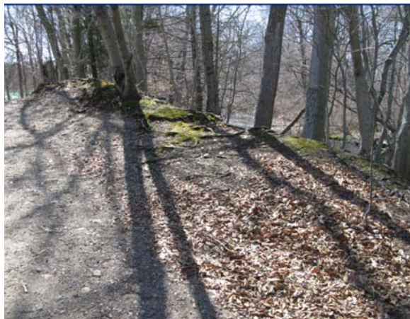
Figure 8. Artificial levee built to a height of 10± feet above flood stage. View taken near south central part of park near a wetland restoration area. Levee continues for about 1000 feet and ends abruptly in a swamp.
