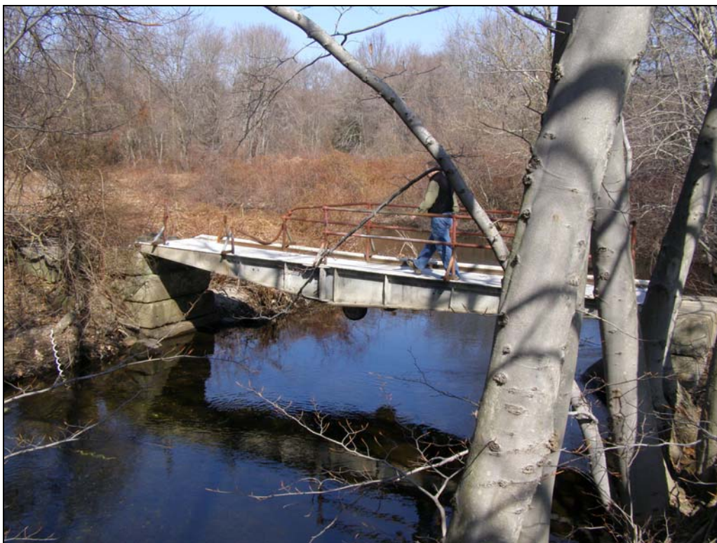
“South bridge” over the Wepawaug River within Eisenhower Park.
