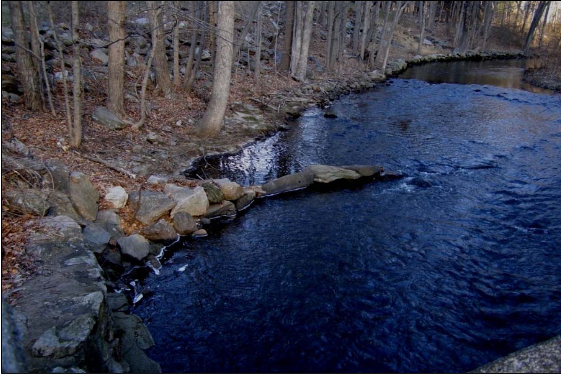
An example of a rock vane.
