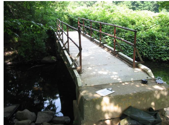
Portable Steel Bridge (south)
