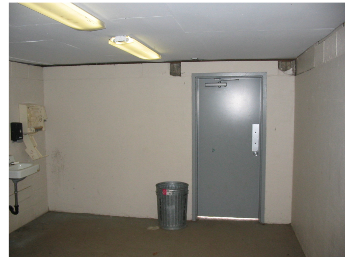
Lower Restroom: interior
