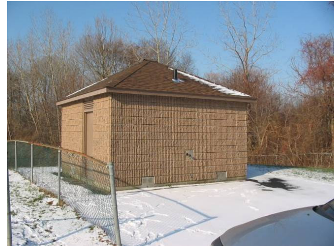
Foote Field Restroom: exterior
