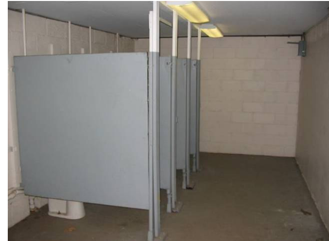
Lower Restroom: interior
