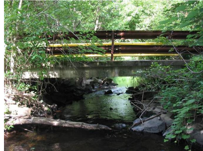
Pre-stressed Concrete Bridge (north)
