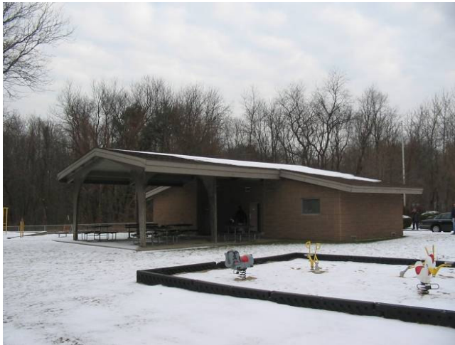
North Street Pavilion: exterior
