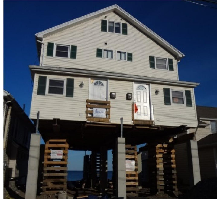
Elevating Homes Protects them from Storm Surge. Hillside Ave Image: activerain.com
