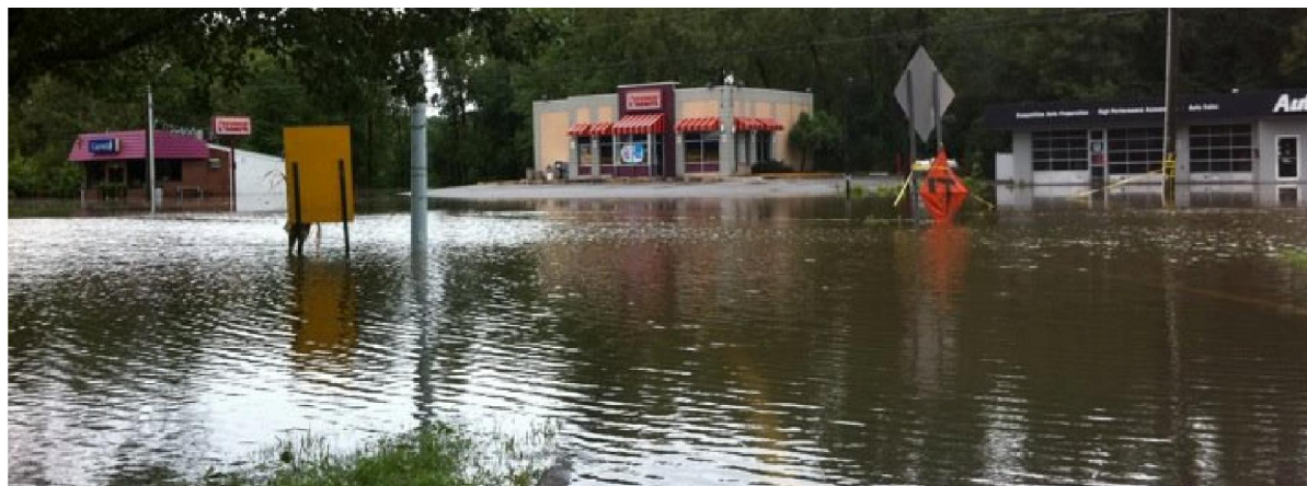
Flooding in Milford after Irene affects business operations Image: Michelle Gervais
