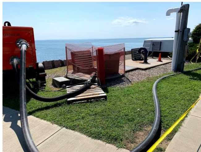
Emergency pump installed at Morningside Pump Station
